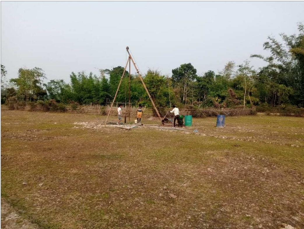
PHOTOGRAPHS SHOWING VIEW OF THE SITE & BOREHOLES UNDER PROGRESS
