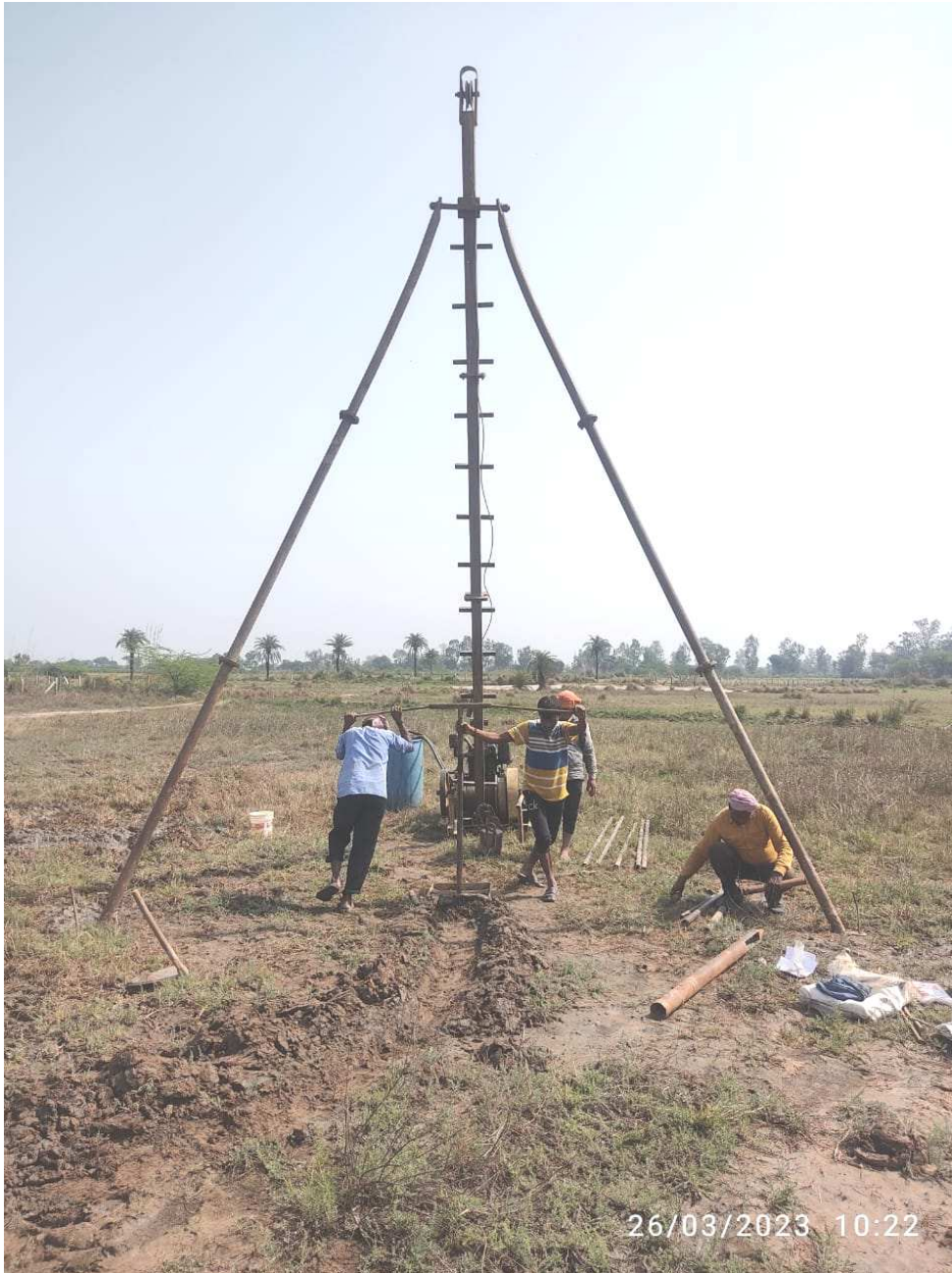
PHOTOGRAPH SHOWING VIEW OF THE SITE & BOREHOLE UNDER PROGRESS
