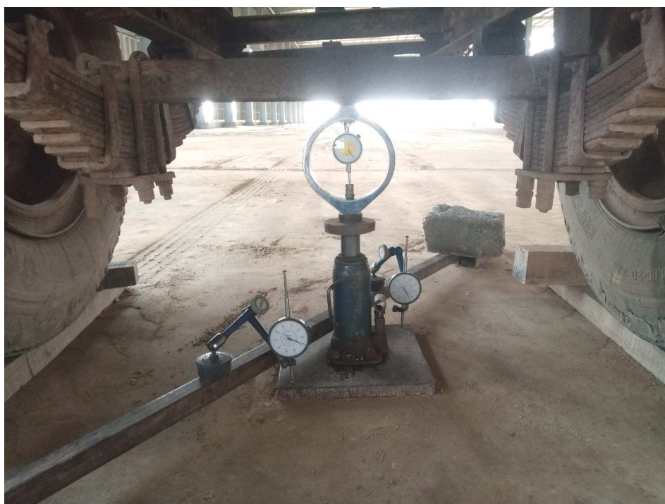
PHOTOGRAPHS SHOWING PLATE LOAD TEST UNDER PROGRESS
